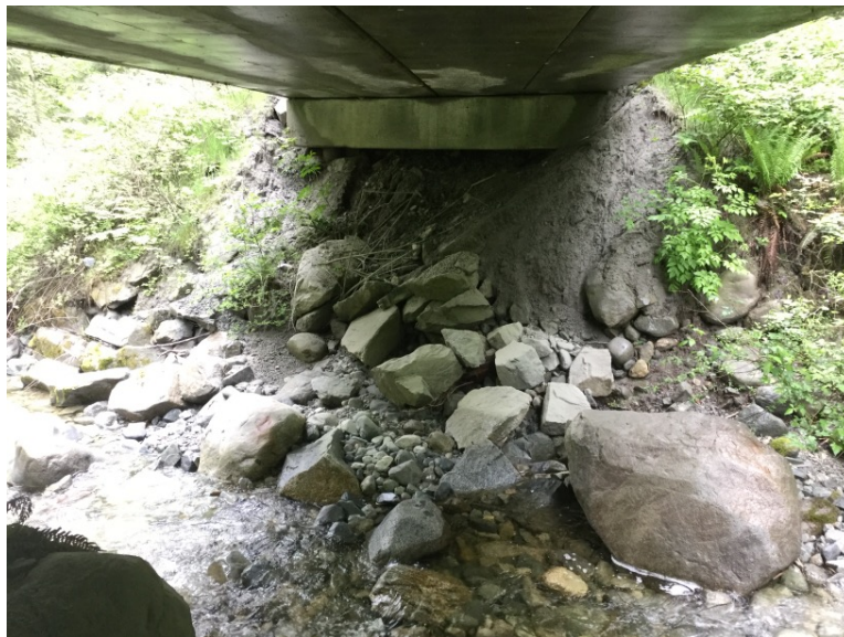
Right Bank Abutment when facing downstream
