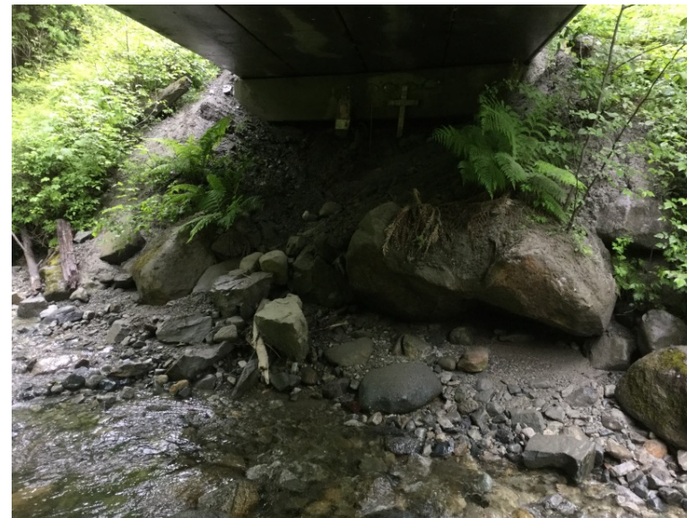
Left Bank Abutment when facing downstream
