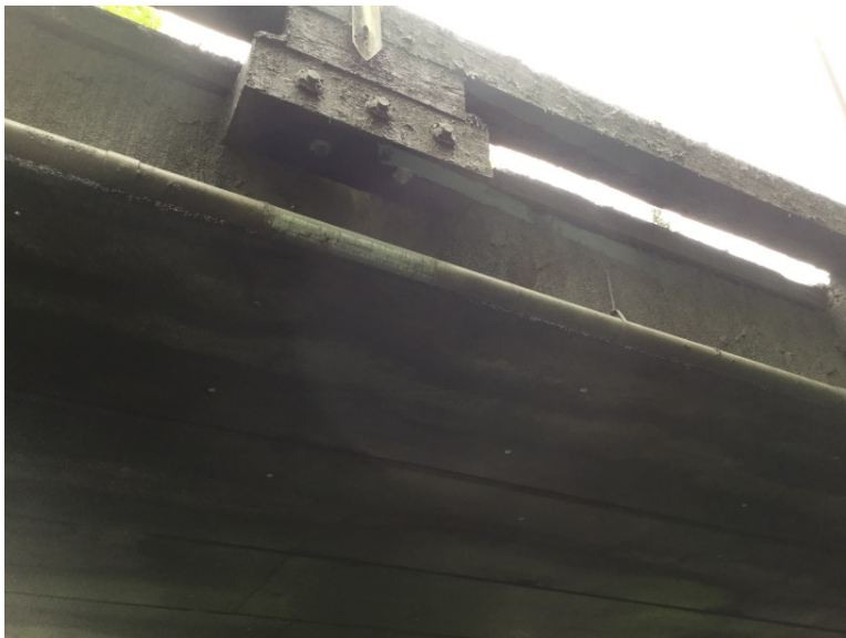
Utilities located at downstream end
